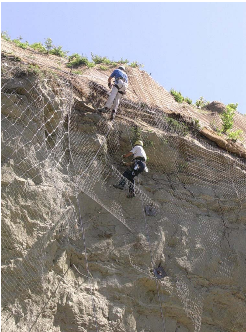
Figure 9.18: Structural engineering measures (rockfall prevention screens) for mitigating hydrogeological hazards at Fontanelice (BO) 14
