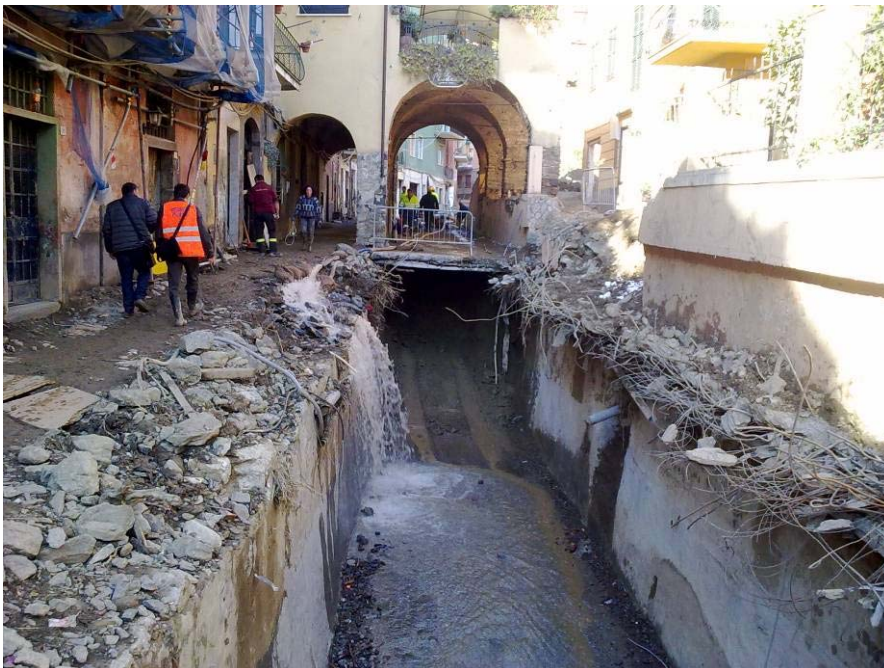
Figure 9.15: Damage to the paving of via Roma (at Monterosso al Mare - SP), beneath which runs the Pastanelli canal 11
