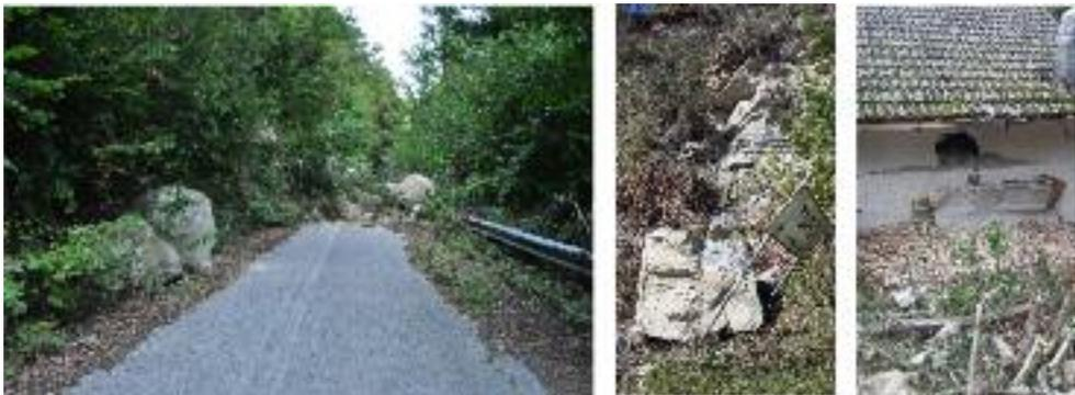
Figure 2: Left: Collapse of blocks that interrupted the road between the Salaria and the village of Tufo (AP); Center: Block collapsed on a road sign at the entrance of Tufo; Right: Wall of a house in Capodacqua (AP) damaged by a block rolled from the overlying slope
